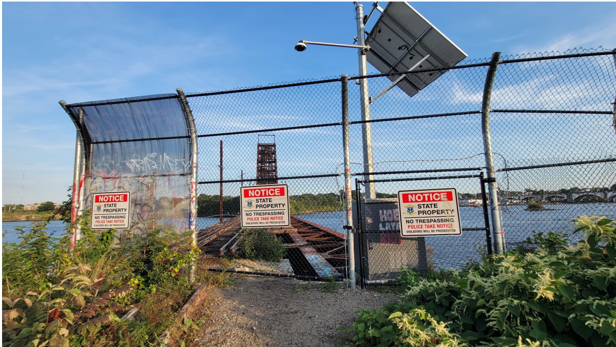
Fence Guarding the Crook Point Bridge
