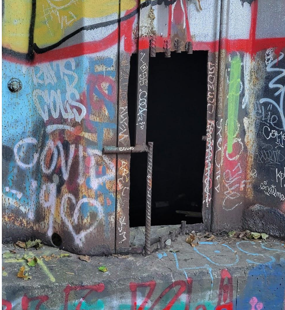
Entrance to the Tunnel, showing the rebar that has been cut away in order to create an entrance
