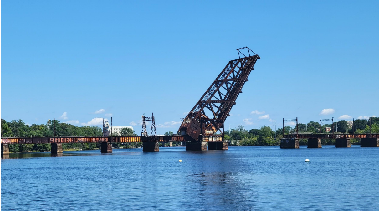
Crook Point Bascule Bridge
