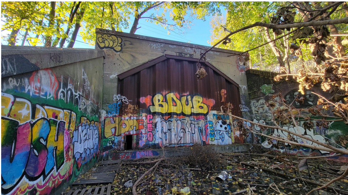
Eastern Tunnel Entrance
